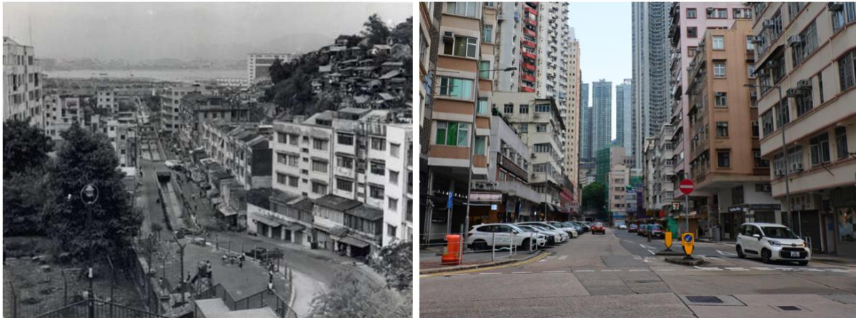
Figure 3: Tai Hang Community Comparison (Left: Historical photograph, Source: Chan, 2016; Right: Current state, Source: Author)
