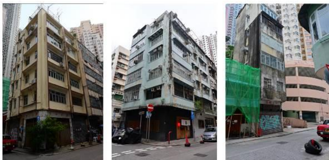
Figure 2: Traditional Chinese Tenement Building ( Tong Lau ) in Tai Hang District (Source: Author)
