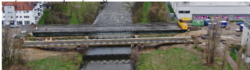
Figure 6 Fully Erected Temporary Bridge
