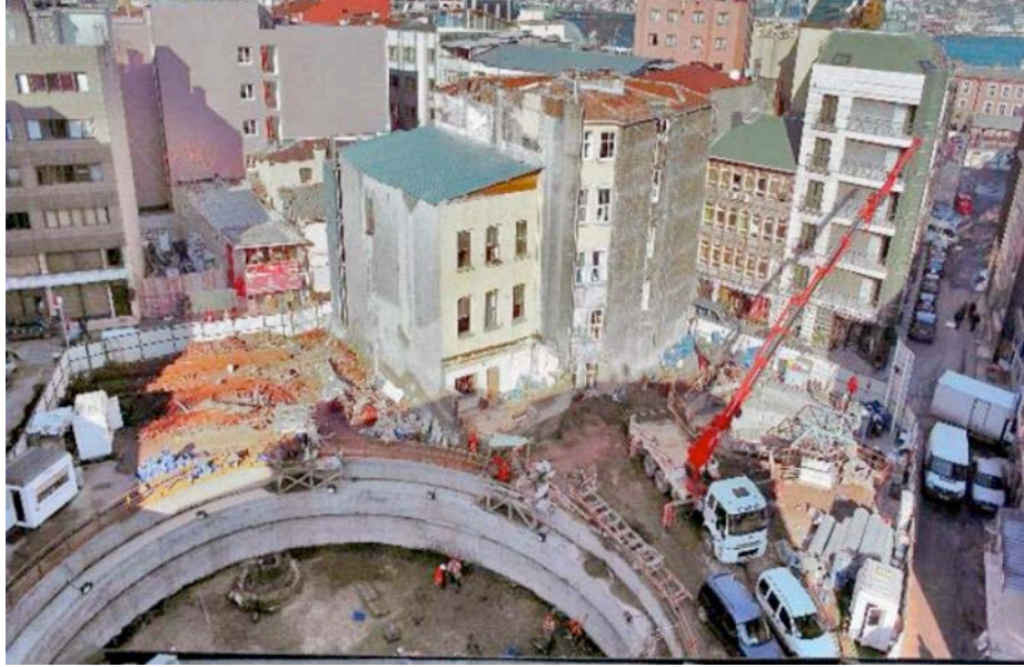
Fig. 7: East shaft (two rings together) (Irmak, 2010: 75)
