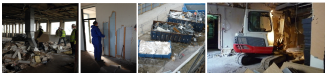
Figure 3: Plasterboard dismantling and segregation in different GtoG pilot projects. From left to right: strip-out activities in London (the UK), manual plasterboard dismantling in Graben (Germany), waste storage in Levallois Perret (France) and mechanical plasterboard dismantling in Brussels (Belgium).
