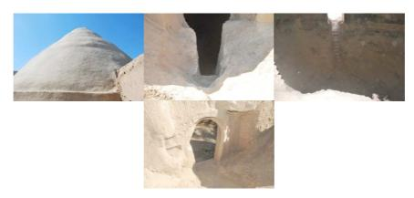
Fig 3. An ice-pit in Kashan, Dome, hatch and ice reservoir are shown, photos by Korsavi.
