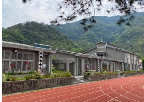
Figure 6: Outside of Classrooms
