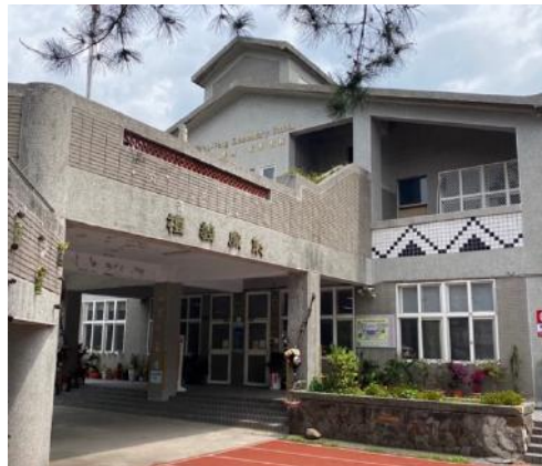
Figure 10: Office Exterior Wall Resource: Taken by the researchers
