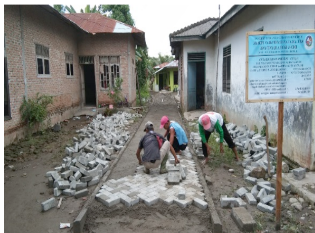
Figure 2: The process of installing paving blocks for the people of Rantang City Village
