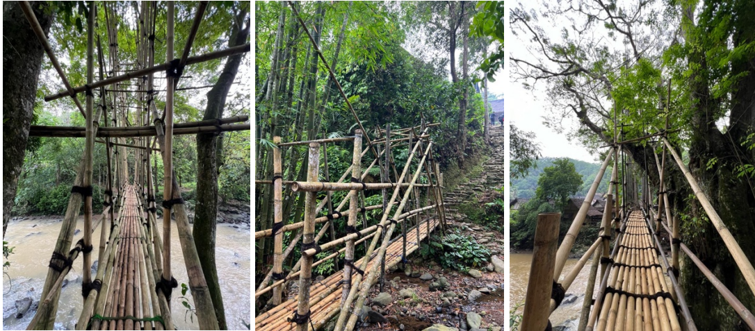
Figure 3: Environmentally Friendly Bridge in Baduy (Personal Documentation, 2023)
