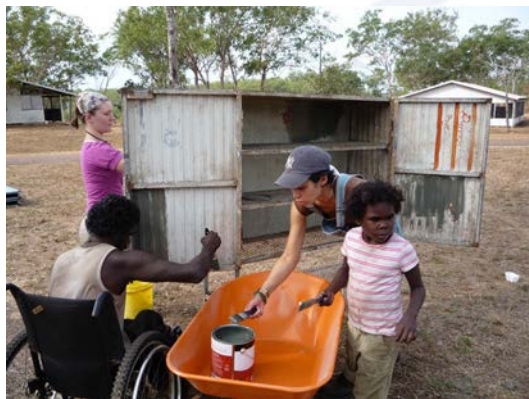
Figure. 3 The wider community enjoyed participating in the construction process.
