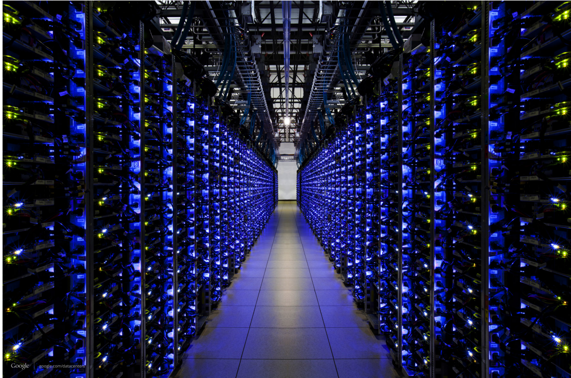
Inside a Google Data Centre, Douglas County, Georgia, USA. (Google, 2014c).
