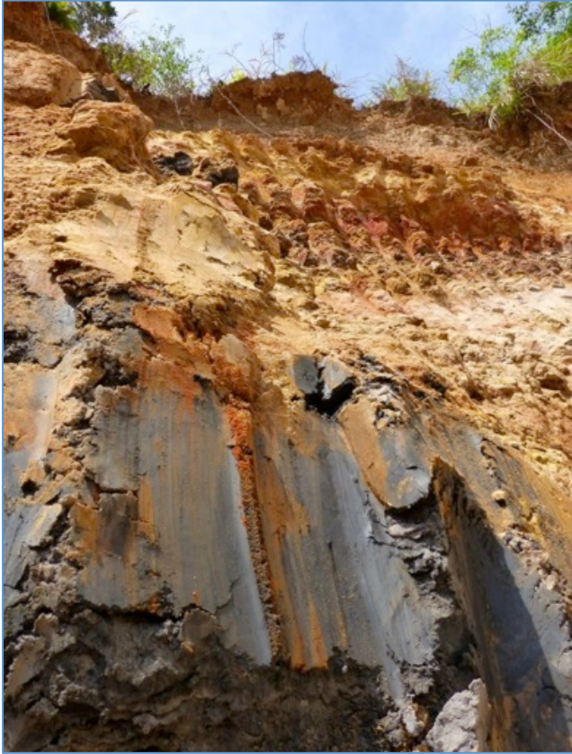
Figure 3: UBD campus clay used for road construction and by Geiger-Ho as material for making various kinds of ceramic art. Similar terracotta clay deposits are used to manufacture ordinary building bricks.
