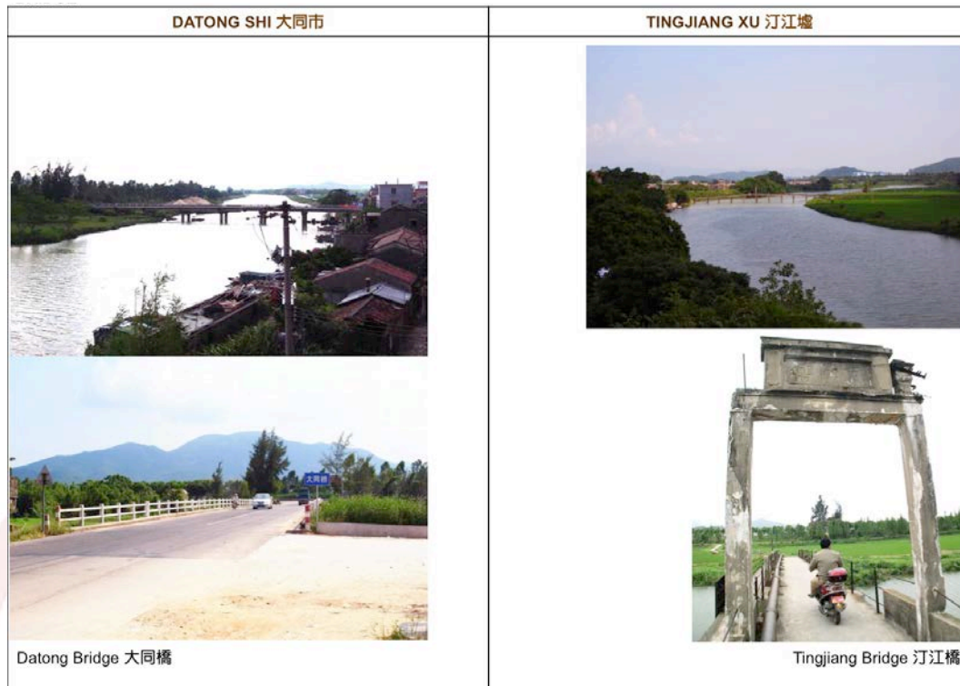
Figure 12. Photos of Datong Shi and Tingjiang Xu: Bridge
