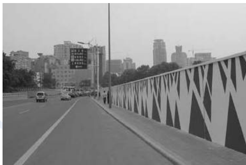
Figure 7: The split to city caused by fence
