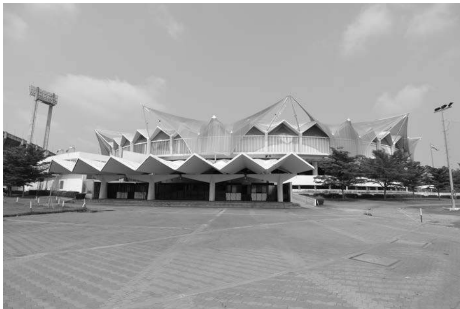
Figure 11. Indoor Stadium Huamark, 1966.
