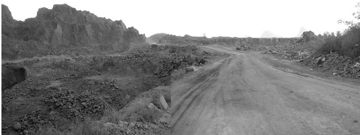
Fig.8- Picture shows excavation site of soil supply for land-filling
