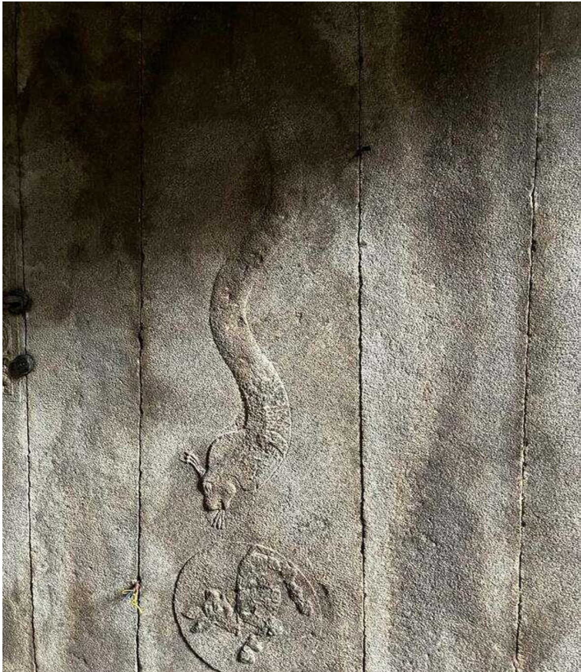
Figure 5. On the roof of the Mandapam in Virupaksha Temple, Hampi (Karnataka) (Image credits- Mr. Amogh Vaidya)
