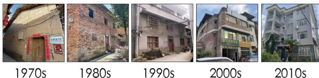
Figure 3: The appearance and characteristics of buildings in different ages in Qingyuan Town Source: drawn by the author
