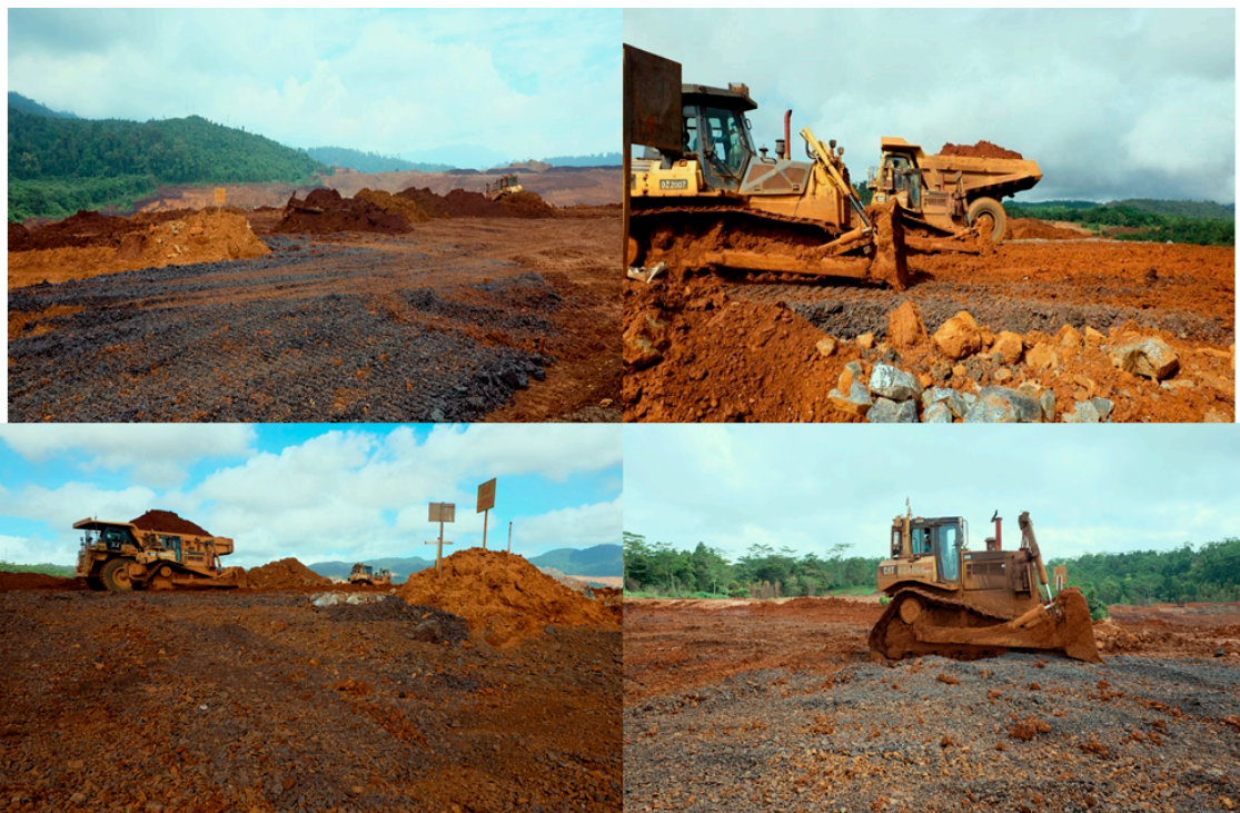
Figure 8: The Use of Slag to Construct Mining Roads
