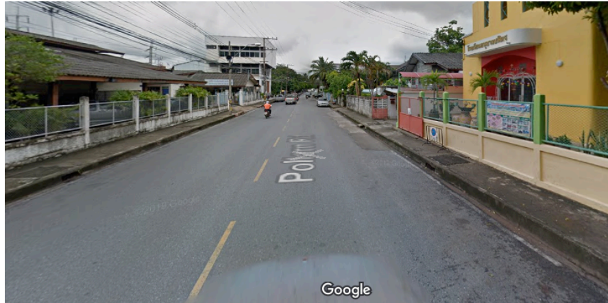
Source: Google Street View Figure3: Lack of protective rail for footpath.
