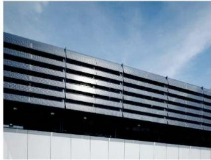
Photovoltaic glass louvers are available in various colors, surface finishes, patterns and coatings to meet specific design requirements.
