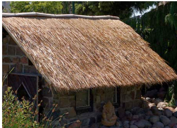
Figure 1. Vetiver roofing.
