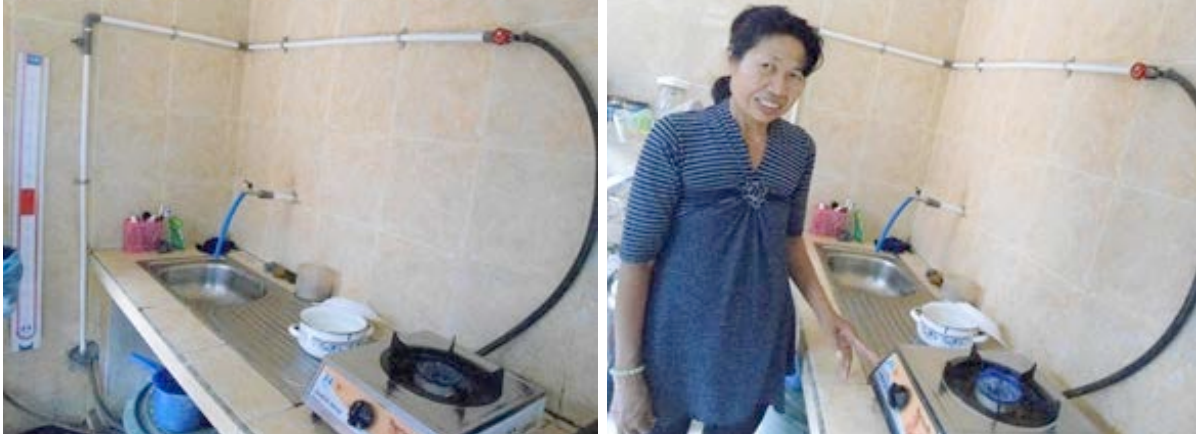
Figure 8: Biogas Installation System (left) and Biogas Product for Daily Usage in Community (right)
