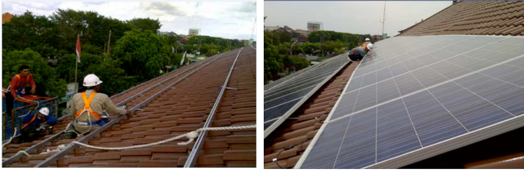
Figure 4: Installation of Solar Cell Panel with Consideration Health and Safety Behaviors
