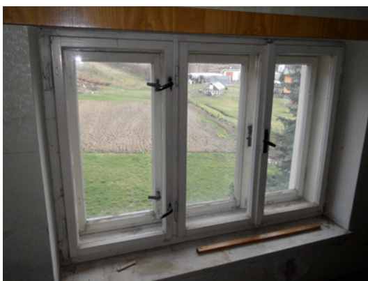
Figure 1: Double casement double-pane window
