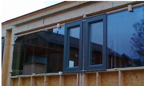
Figure 7: Opening and fixed window.
