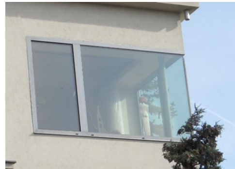
Figure 8: Window with integrated casement frame.
