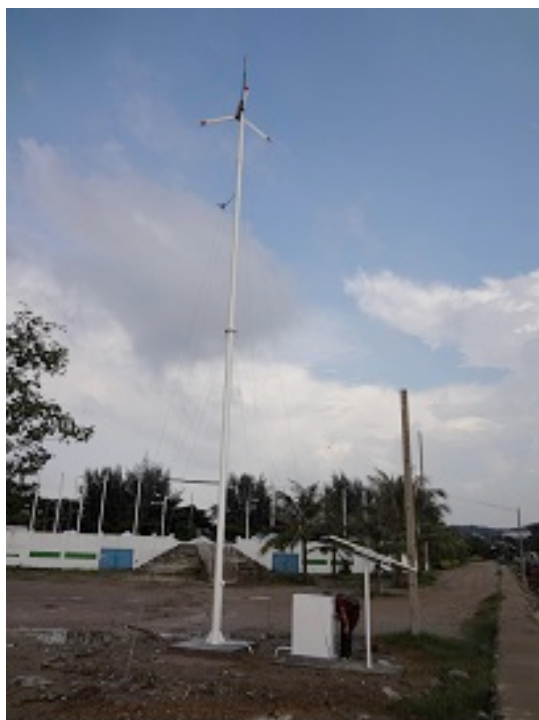
a) Complete installation
