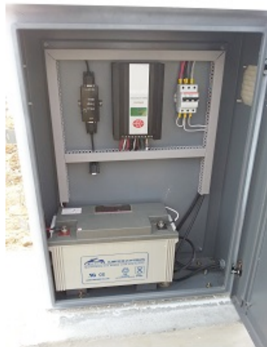
b) Equipment within the cabinet
