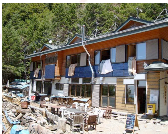
Fig. 1 Natususawa mountain lodge at 2,000m. Solar panels and small wind turbines are seen.
