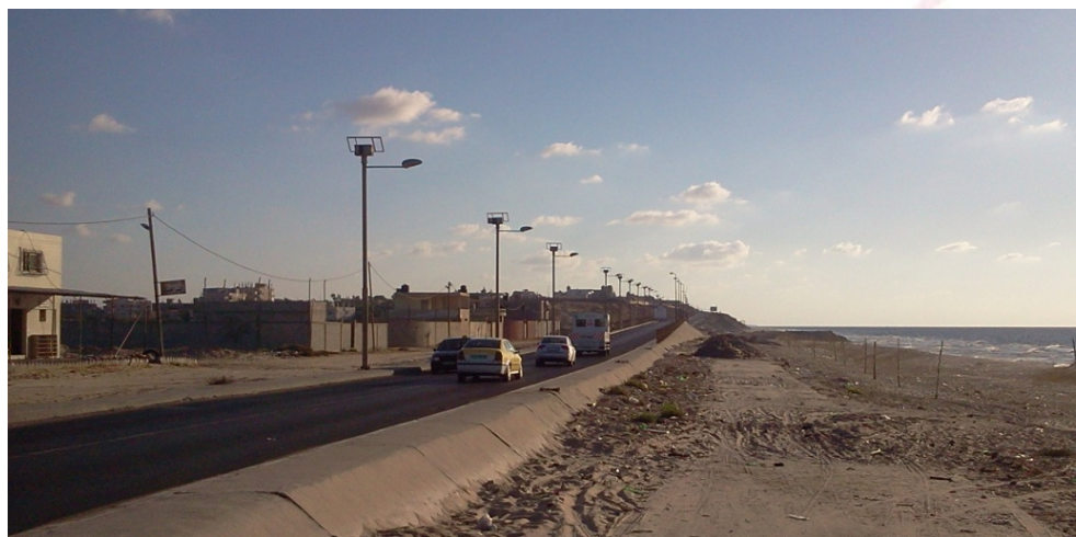
Fig.6 PV Street Lighting System at the Valley of Gaza
