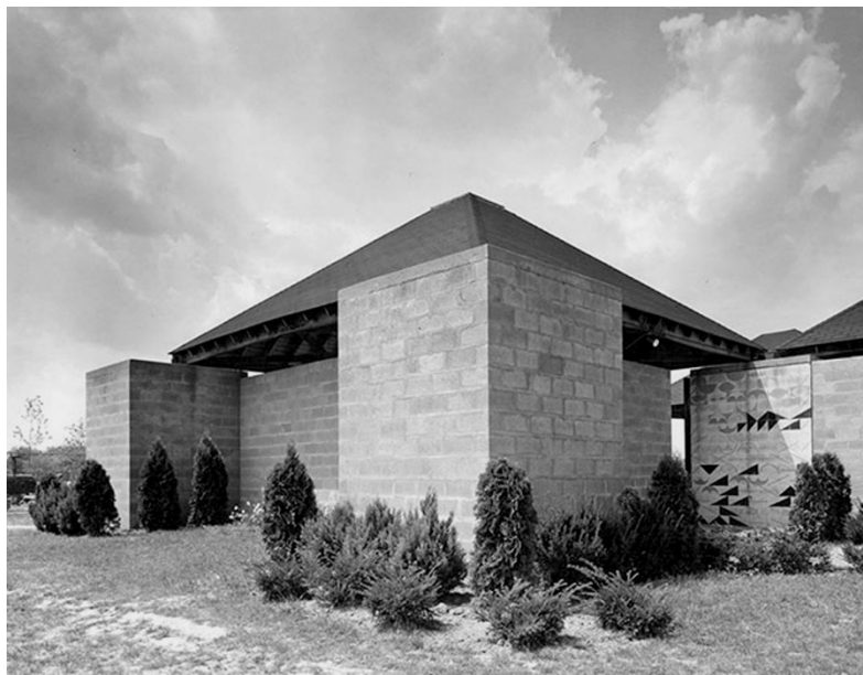
Figure 8: Trenton Bath House (1954-55). Source(s): Brownlee and De Long 1991.
