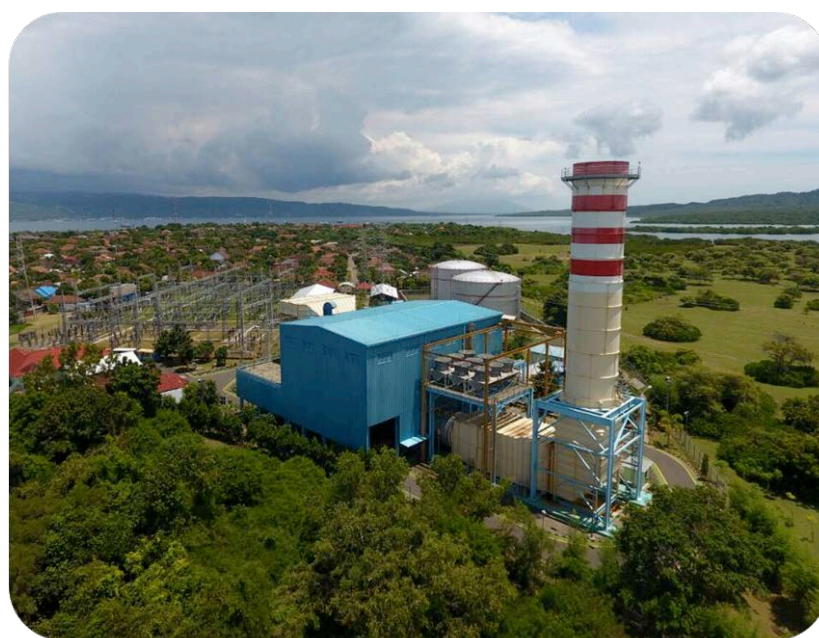
Figure 1. Appearance of Gilimanuk Gas-Turbine Power Plant in West Bali [Purwakanta, I.N., 2017]
