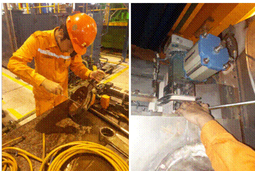
Figure 5. Activity of Re-Design Waste-Gate Valve: (left) Dismantling the Waste-Gate Valve in PLTDG 10 Pesanggaran; (right) Assesmbly the Re-Designed Waste-Gate Valve in PLTDG 10 Pesanggaran.
