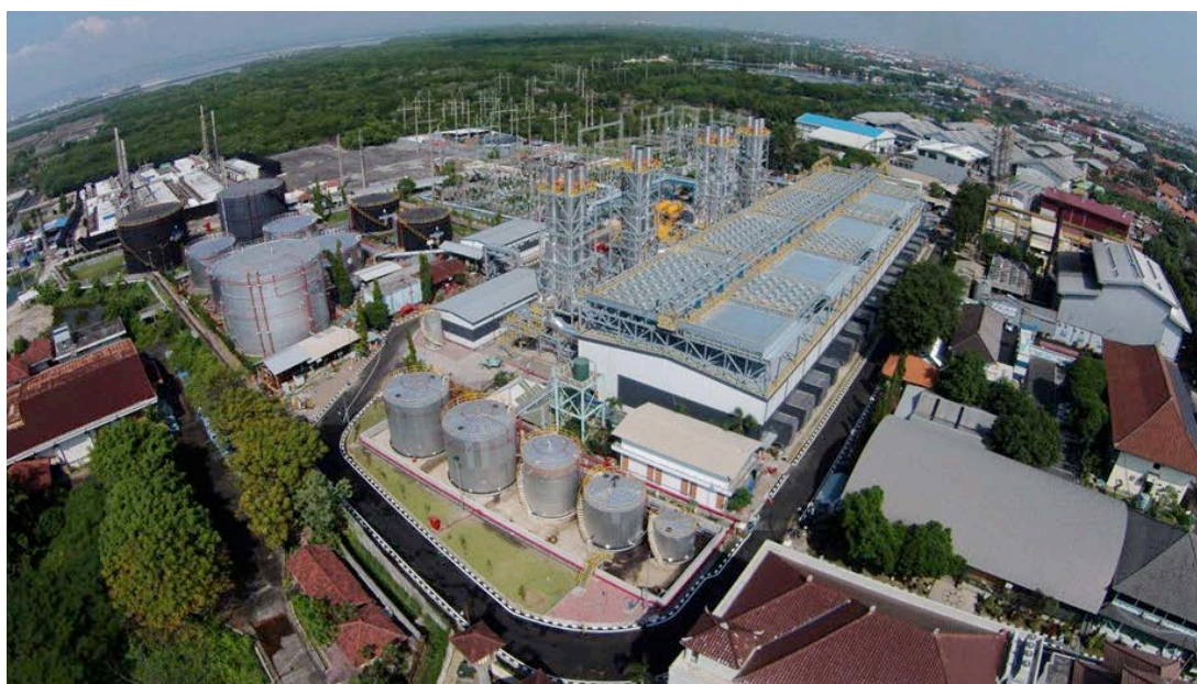
Figure 1: Overview of Pesanggaran Power Generation, Bali Province, Indonesia. It operates by PT Indonesia Power UP Bali, a subsidiary of State Electricity Company (PT Perusahaan Listrik Negara – PLN Persero), with main core business in operation and maintenance of power plant [Subawa P., 2016].
