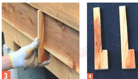
Fig.10-1 Text (Using a jig for siding)
