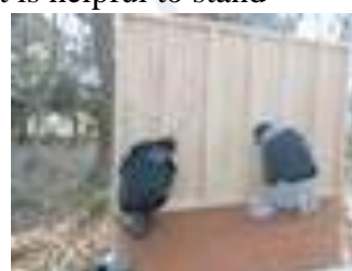
Fig.4-2 Structural frame and plywood together form a wall
