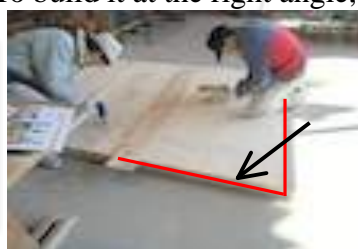
Fig.4-2 Structural frame and plywood together form a wall
