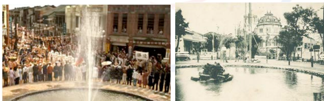
Figure 7 Rebuilt fountain roundabout (Left Figure); Fountain roundabout in Japanese colonial period (Right figure)
