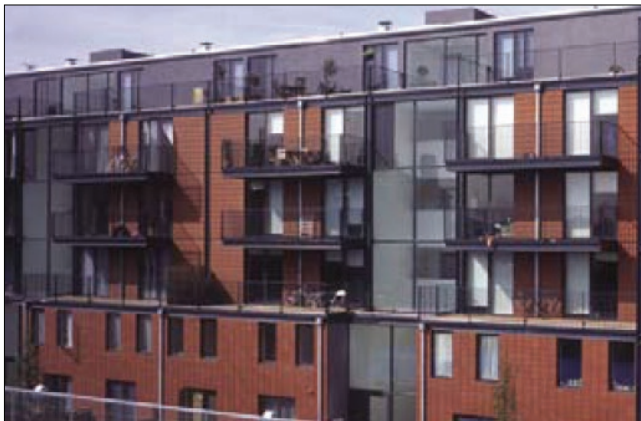
Fig. 2: The use of steel construction in a social housing project, UK (Lawson, 2009)
