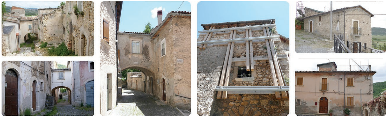
Figure 1. Views of the medieval village of Caporciano. The aggregate consists of approximately 300 buildings, with its traditional architecture of rural type, consisting mainly of vertical walls (coinciding with the elevated structure) in local stone, with rustication and gravel of various sizes, which can reach 90-100 cm thick, even with small-recovered brick elements. The village has an outer belt of expansion characterized by newer buildings (from the 50s onwards), with concrete-frame technology and plugging in semi-solid blocks of brick or masonry bearing.
