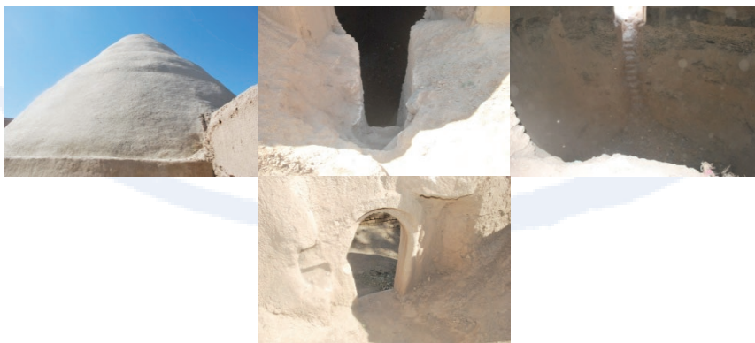
Fig 3. An ice-pit in Kashan, Dome, hatch and ice reservoir are shown, photos by Korsavi.
