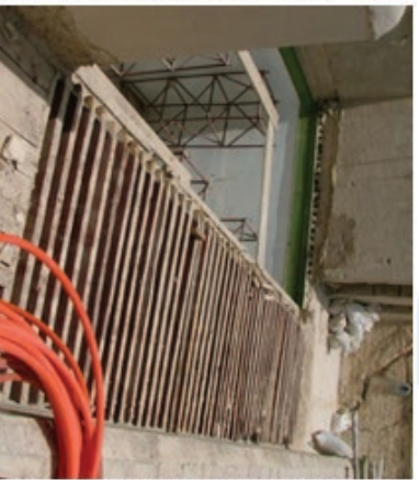
Restoration work in Riad, Laroussa roof, Fez, Morocco
