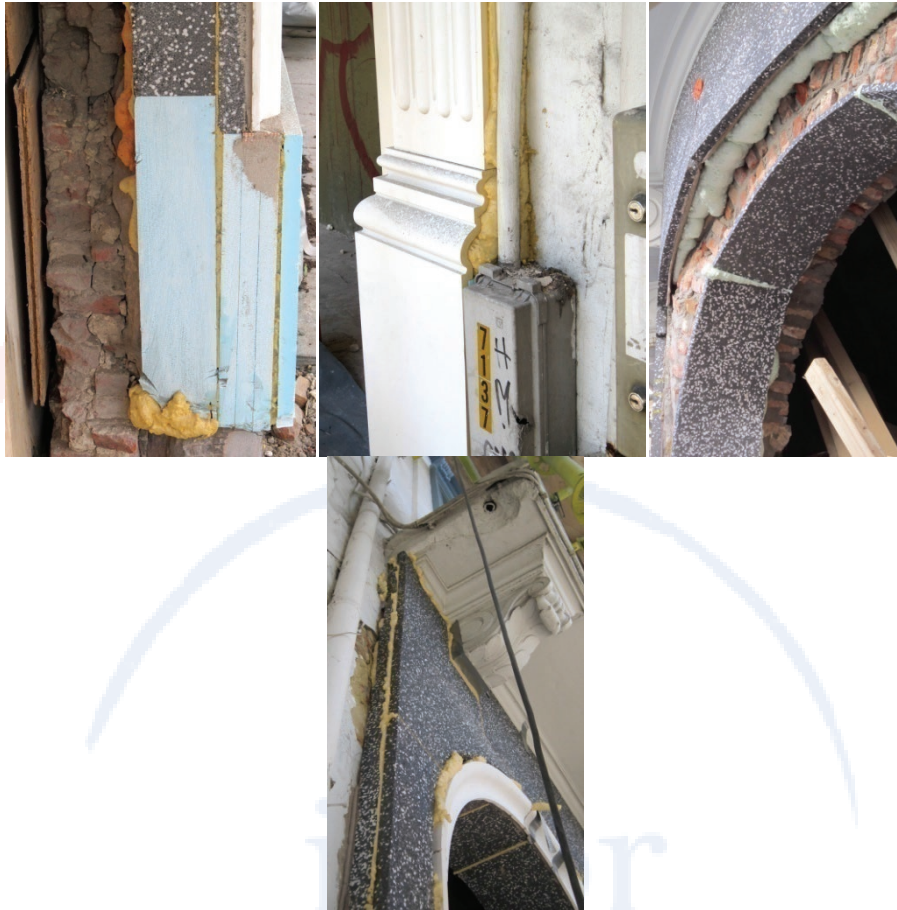
Image 5. 1, Building envelope insulation; Details; Building in Antwerp 2013
