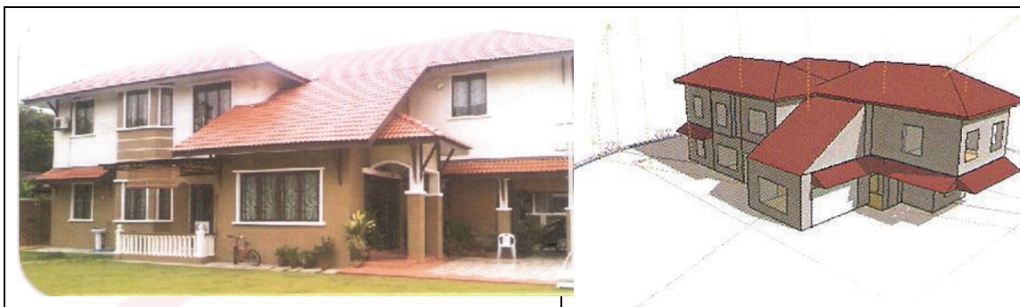
Figure 2: The selected existing house in Malaysia for Ecotect environment analysis (Source: 1 st year group work report: Passive Design Strategies for a House, AAR 1297 Environmental Science System, 2012/2013).
