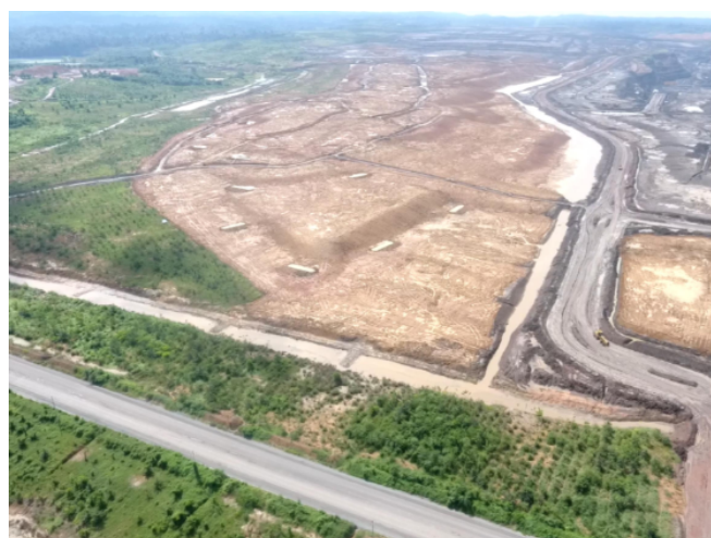
Figure 6: Drainage system in IMM Mine Site
