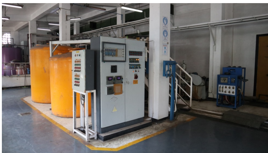
Figure 6: Reverse Osmosis Conversion Coating Unit SHT
