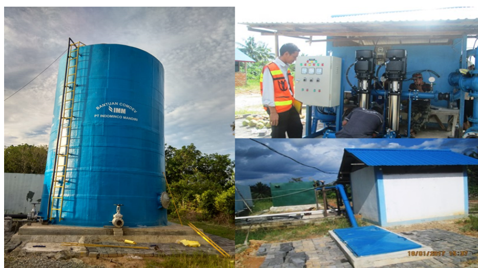
Figure 5: Water Treatment Plant Installation Activities
