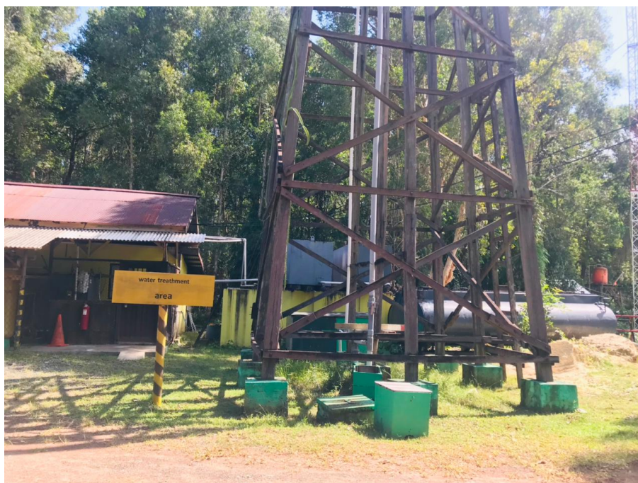
Figure 5: Processed Water Utilization from MHP for Domestic Needs
