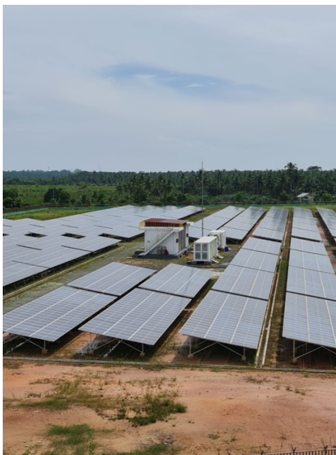
Figure 3: 3 MW Solar Farm IMM
