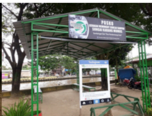
Figure 2: Post of GMSS SKM located on Abdul Mutholib Street.
