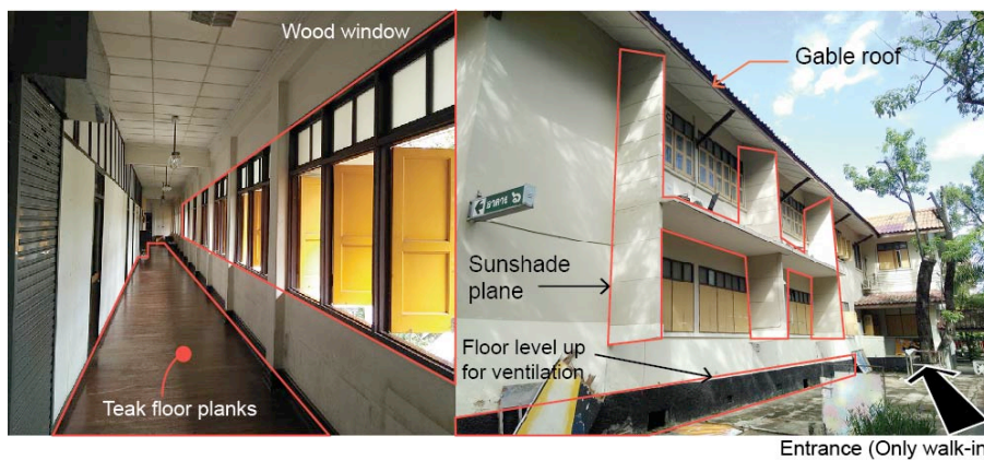
Figure 3: Digital Photo of Building at the interior and frontal view.
