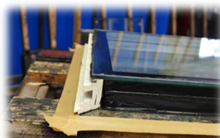
Figure 12: Section of wooden window with a low frame
