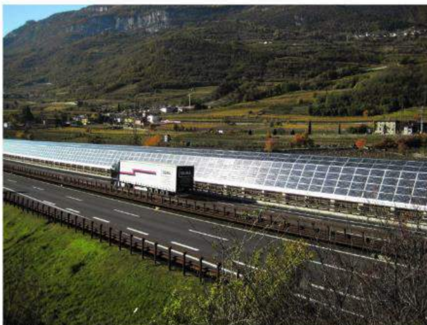
Figure 2. integrated photovoltaic system in the highway guard-rail. Autostrada del Brennero IT. source: www.autobrennero.it
