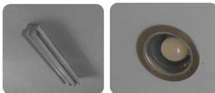
Figure 5: 100 Watt Tubular Lamp (left) Replacement to 9 Watt Light Emitting Diode Lamp (right) Around Main and Supporting Building
