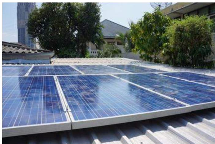
Figure 5: Photovoltaic system on the rooftop of a sample house.
