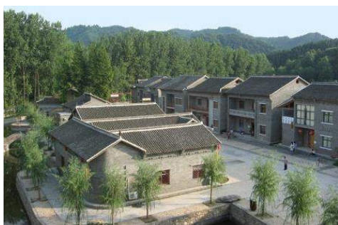
Fig.5 Eco-building in yanhe new village
