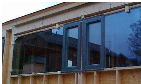
Figure 7: Opening and fixed window.
