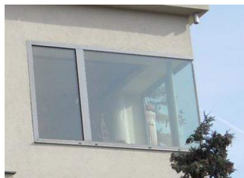
Figure 8: Window with integrated casement frame.
