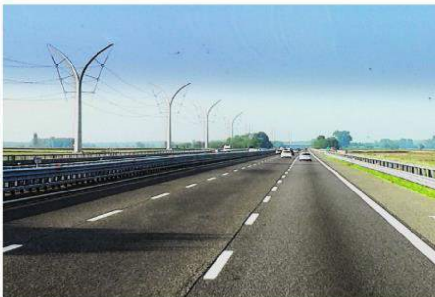
Figure 7. Power lines near Bereguardo IT. Photo of the author (© G. Pozzi).
