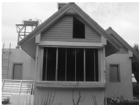
a. South façade of the test building
