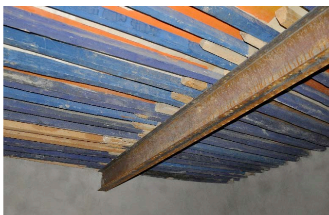
Figure 5: A Steel Beam in an Auxiliary Room. Photograph by Author
