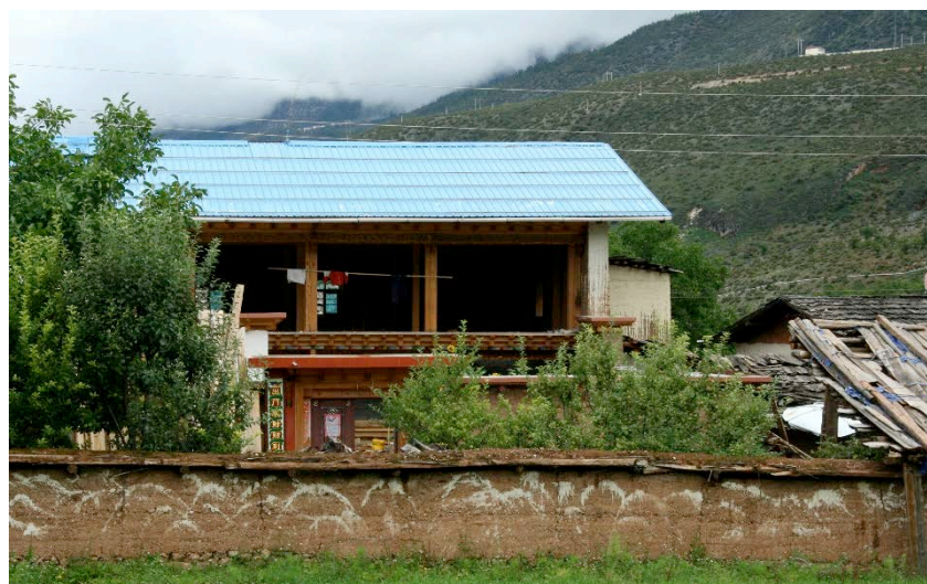
Figure 3: Sloping Roof Made of Colored Steel Tiles in Newly Built Tibetan Houses. Photograph by Author
