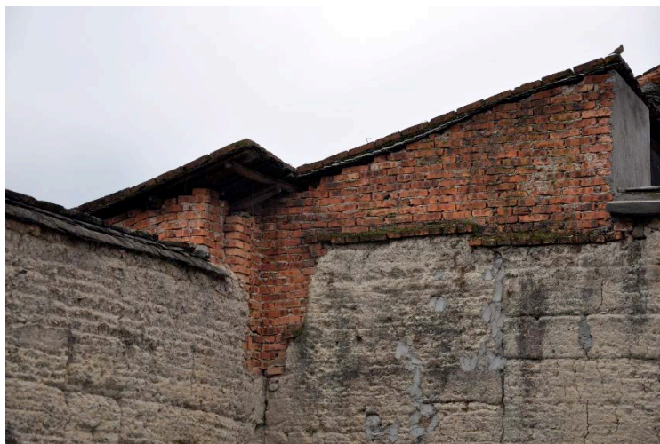
Figure 8: The Added Red Brick Wall Juxtaposes the Original Rammed Earth Wall. Photograph by Author
