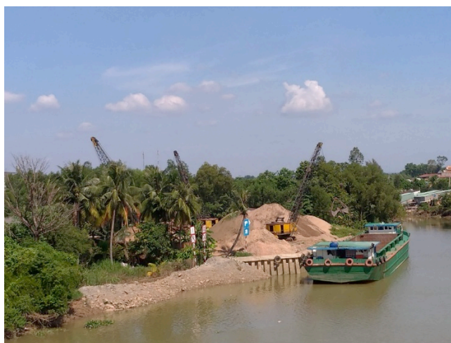
Figure 14: Sand mining activities just below the bridge
