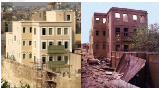
Figure 8:A picture shows intermediate step for (AL-darb AL-AHMAR) development project done by the aghakhan authority.
