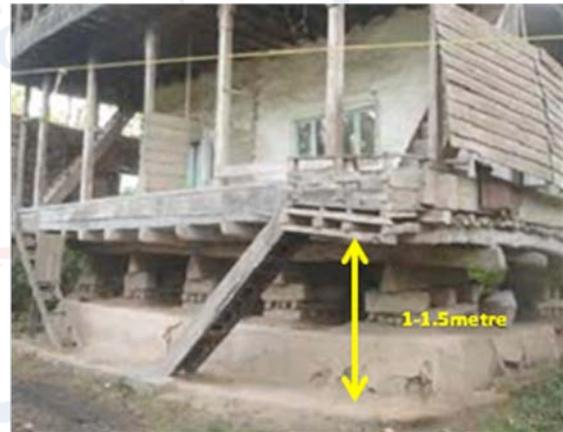
Fig(5): the height from the ground
