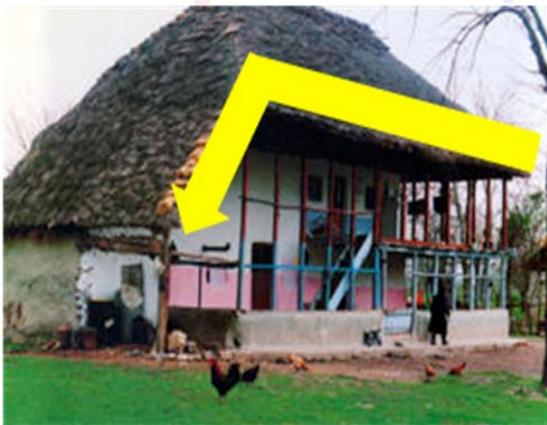
Fig (4): long chimney protected building from curved rains or strong winds
